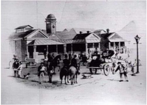
The first official Post Office built on the corner of Bourke Street and Elizabeth Street
